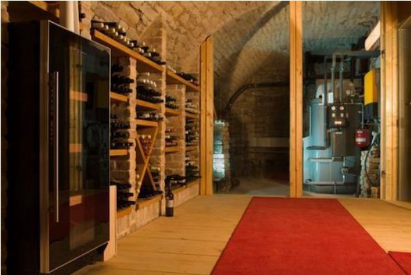
Vaulted cellar with plant room
